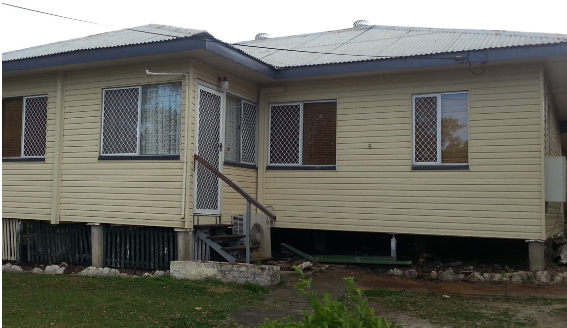
Before and after of guttering works.
